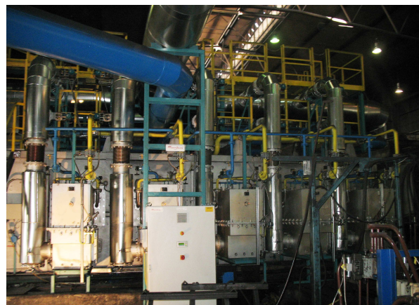
Fig. 8. Furnace sidewall installation - HRS burners
