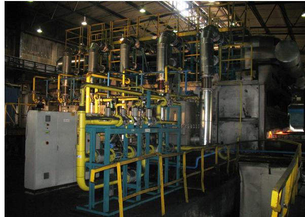
Fig. 16. Furnace and combustion system after revamping
