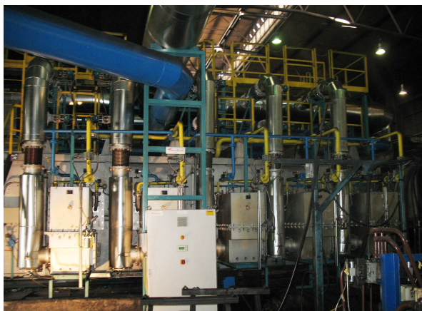
Fig. 15. Furnace sidewall installation - HRS burners
